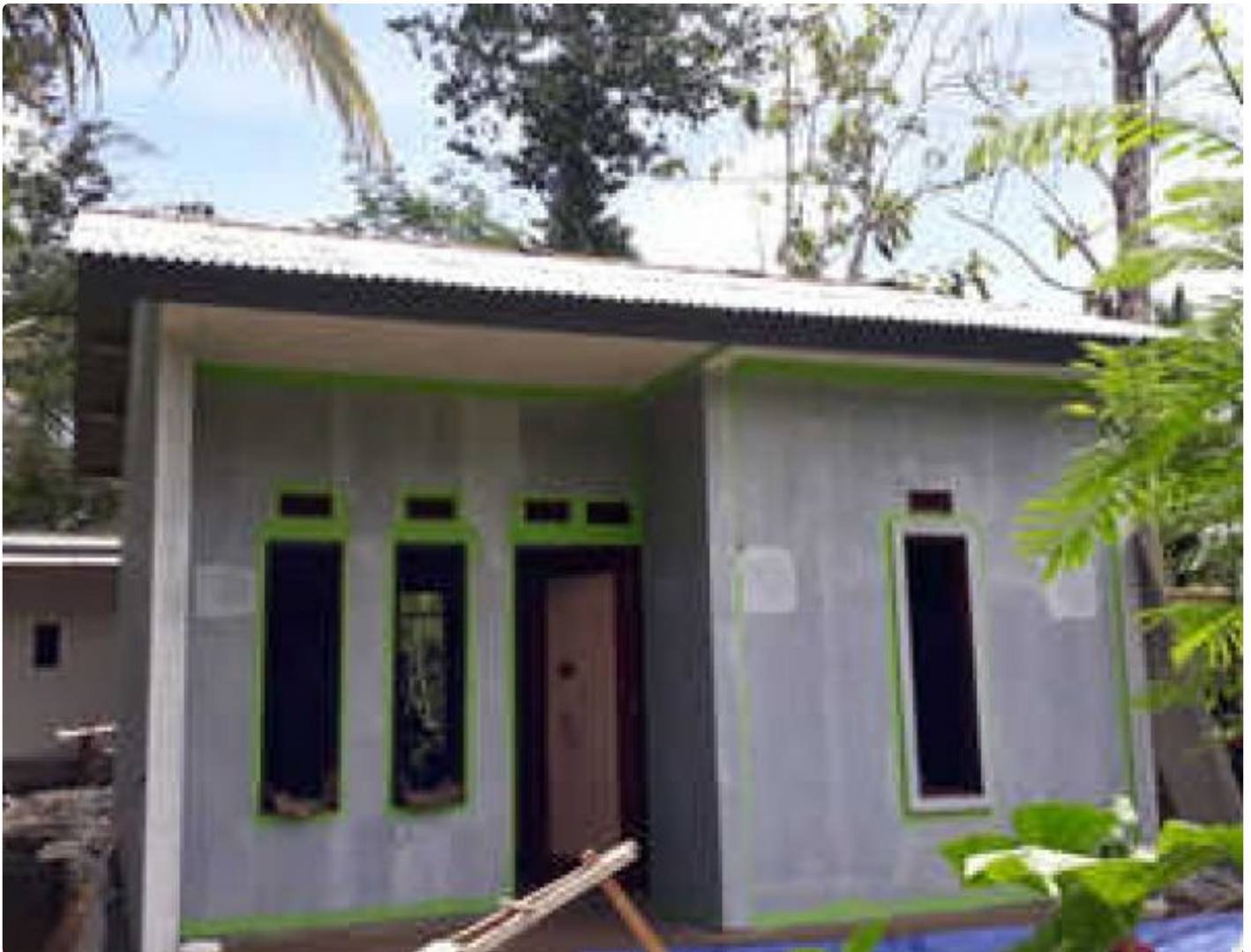
RTLH program TMMD selesai tergarap
